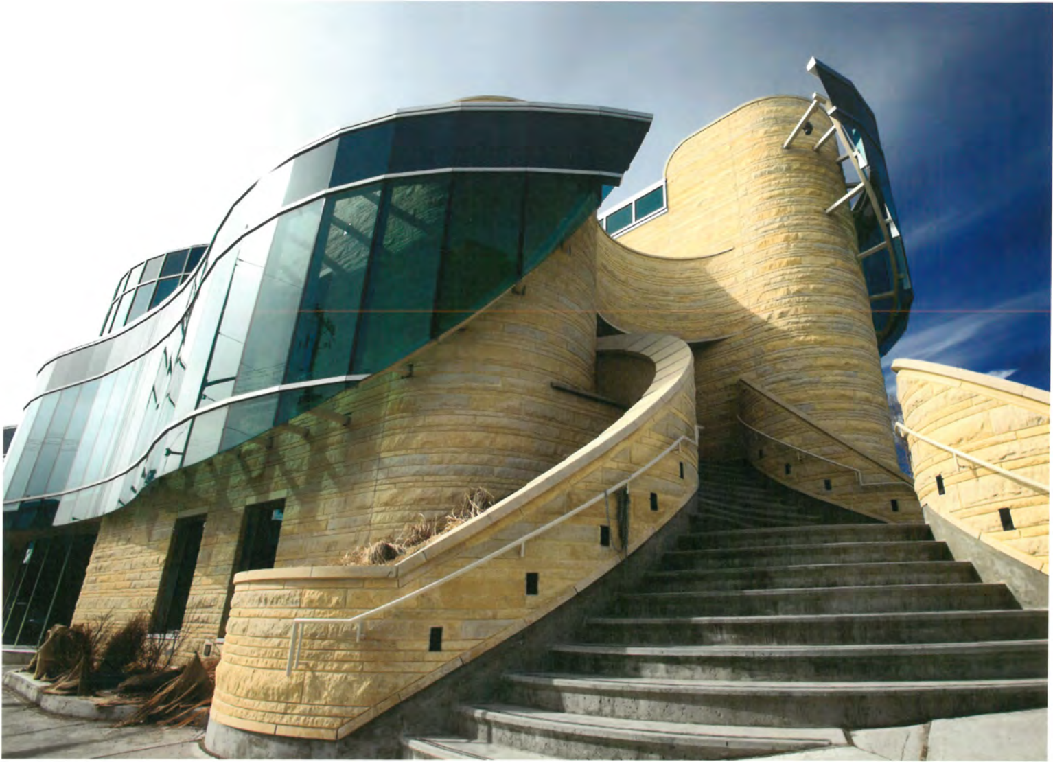
Wabano Centre for Aboriginal Health first opened its doors in 1998 on Montreal Road in Vanier. The award-winning centre, which was redesigned in 2013 by architect Douglas Cardinal, his son Bret Cardinal and Mark Conley, provides holistic health services to the Ottawa First Nations, Métis and Inuit population. The 25,000-square-foot expansion includes new meeting spaces for community groups, outreach and after-school programs, crisis intervention initiatives and workshops showcasing Indigenous art and culture.
